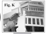
☐ Secure fascia boards with screws, make sure that spacing between fascia boards is even at rafter ends. (as shown Fig. K, glue end caps in place at this
