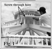
Hold roof panels in place with screw & cap through roof panel channels into roof panels (Fig. I)
