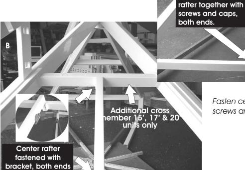
Fasten center rafters to brackets with screws and caps both ends.
